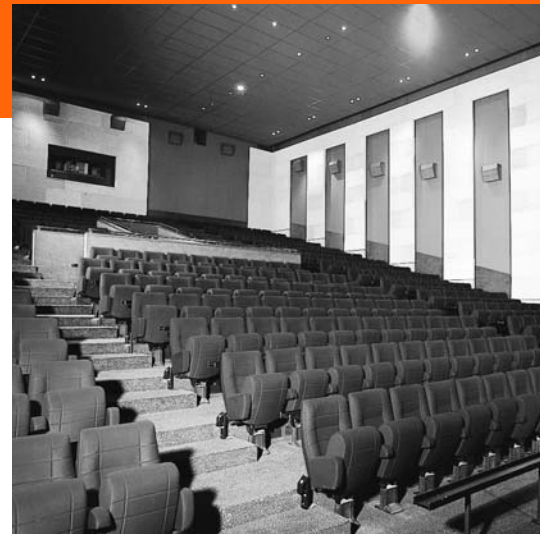
Cinema auditoria are steeply raked to provide a good view of the screen from every seat. This inevitably means very high walls.
