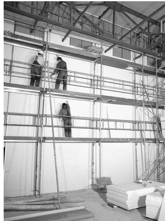
Despite their small cross-section, FERMACELL partition walls meet all structural safety requirements even at heights of nearly 10 m.
