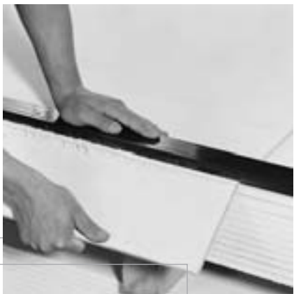
Snapping off a scored section of board
