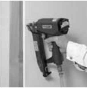
Fixing the boards on a timber subframe with staples
