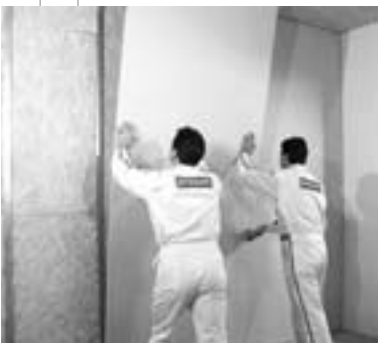
Mounting the boards on a timber subframe
