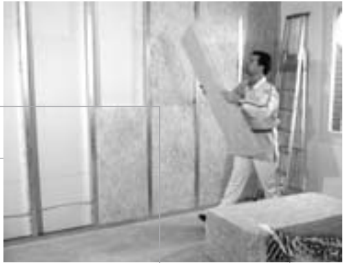
Installing mineral wool insulation batts
