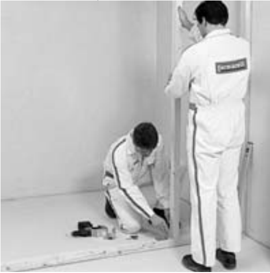
Installing timber studs
