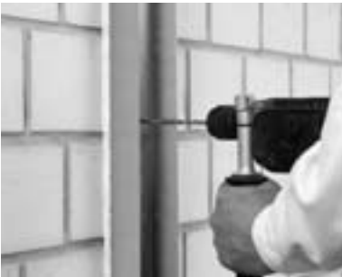
Fixing C studs to the walls
