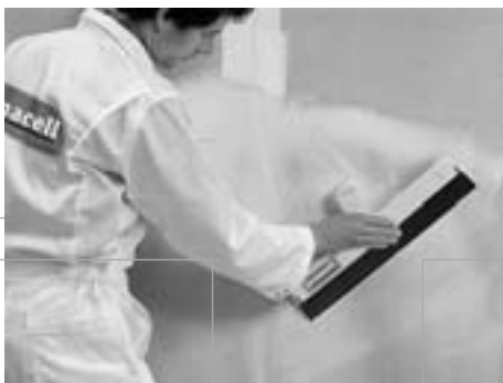
Fine Surface Treatment (semi-gloss finishes)
