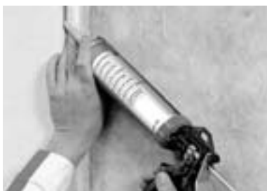
Jointstik is applied to the edge of the board
