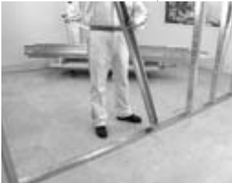
Fitting the C studs in place
