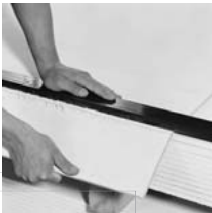
Snapping off a scored section of board
