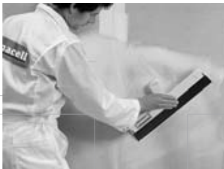
Fine Surface Treatment (semi-gloss finishes)
