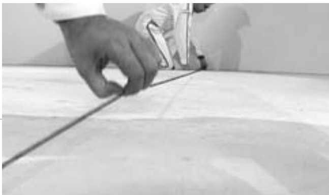
Setting the position of the partition with a chalk line
