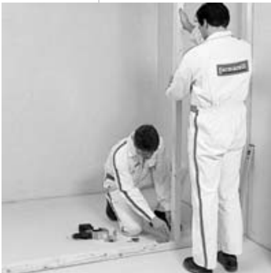
Installing timber studs
