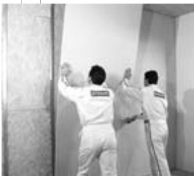
Mounting the boards on a timber subframe
