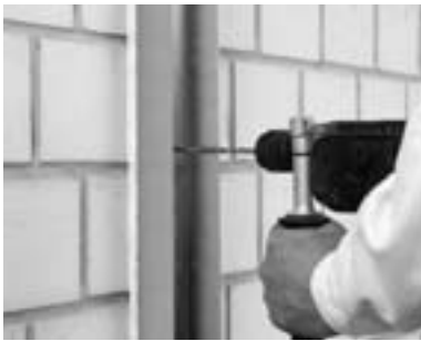
Fixing C studs to the walls
