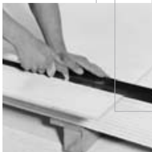
Scoring a board using FERMACELL board knife
