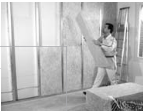
Installing mineral wool insulation batts
