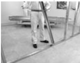
Fitting the C studs in place
