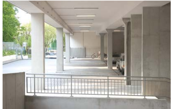
Ceiling insulation above entrance to large garage
